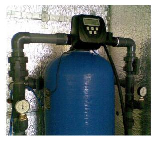
mimics what happens when untreated dissolved iron comes into contact with the air. Within the treatment system the dissolved iron precipitates in the first tank and is carried into the second tank where it is filtered in a Pyrolox, Birm or multi-media filter. Chlorination and ozonation can also be used as an additive in the removal of iron.
